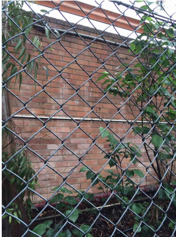
Photograph 2 – Brick masonry wall along Hope Street
