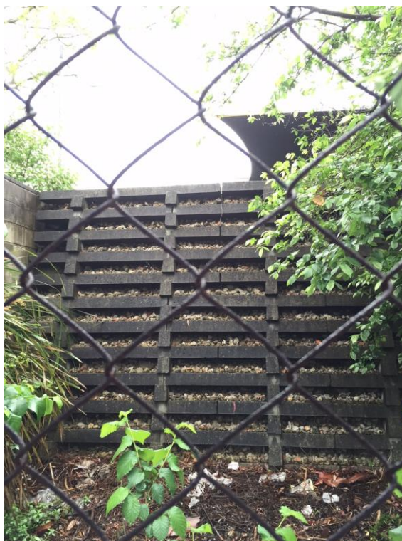
Photograph 4 – Concrete crib wall
