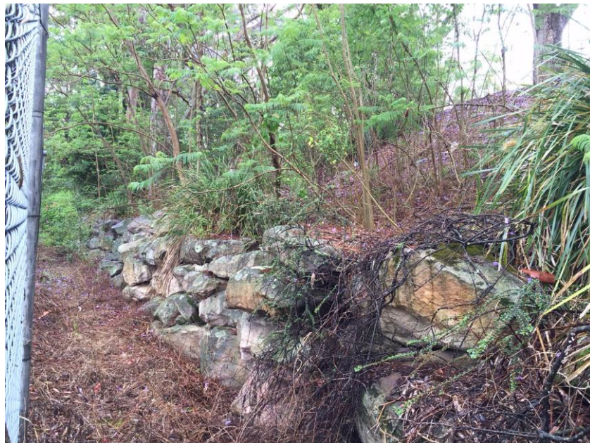
Photograph 3 – Sandstone block wall
